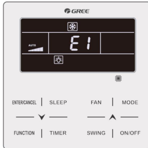
Power-on High-pressure Protection Fault Interface
