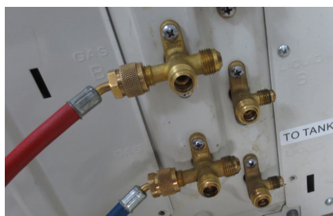
Installation of rubber hose
