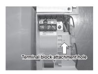
Attach terminal block ① using screw② in the direction shown in the figure.
